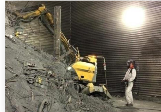
Photo: AB SVAFO. Demolition of biological shield, research reactor in Studsvik.
